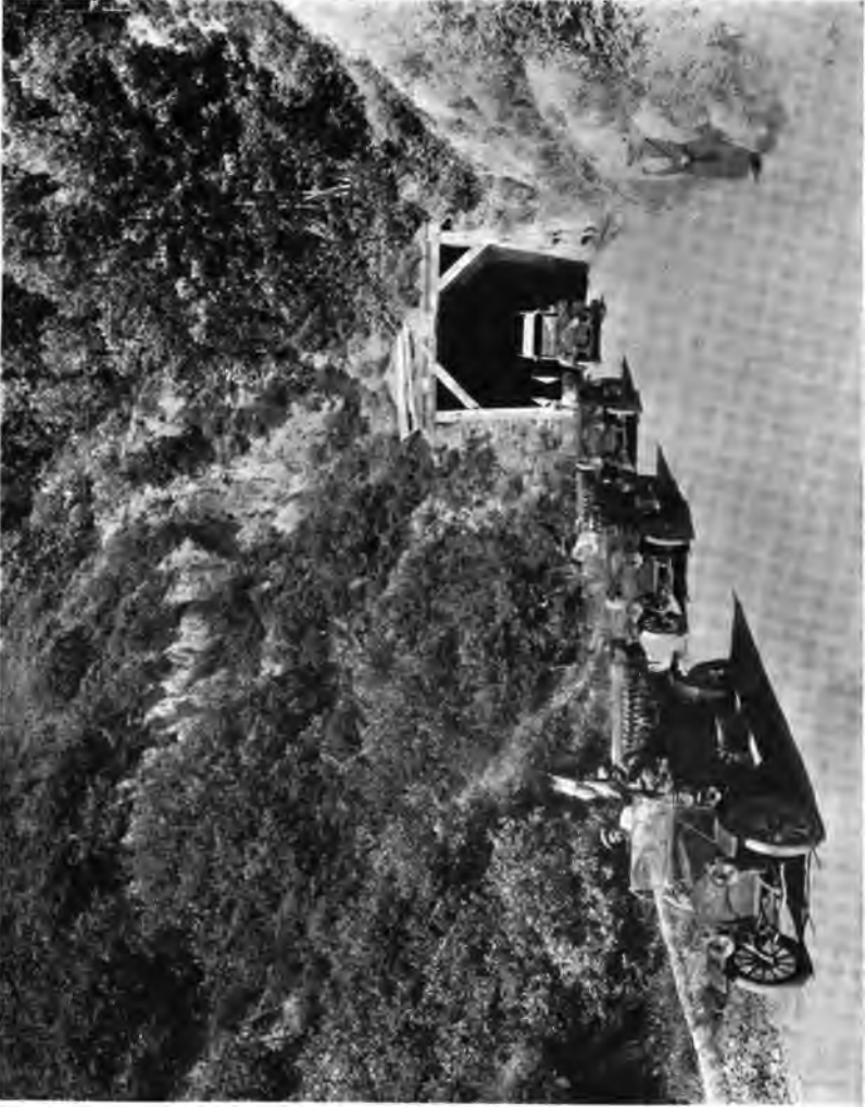
The tunnel connecting Alameda and Contra Costa counties, built by joint action of the Boards of Supervisors.
